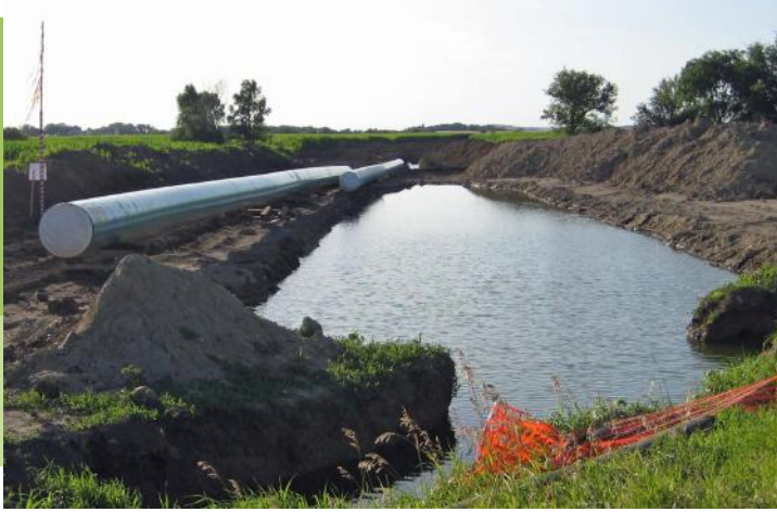
Construction of the first Keystone Pipeline near Yankton, SD
